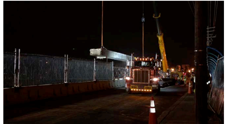
Concrete Beam Removal - Night
