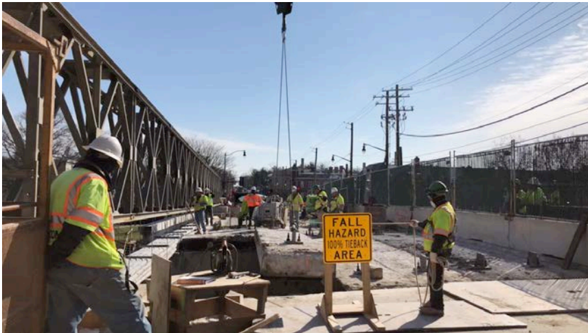
Concrete Beam Removal - Day
