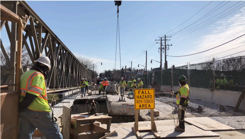
Concrete Beam Removal - Day
