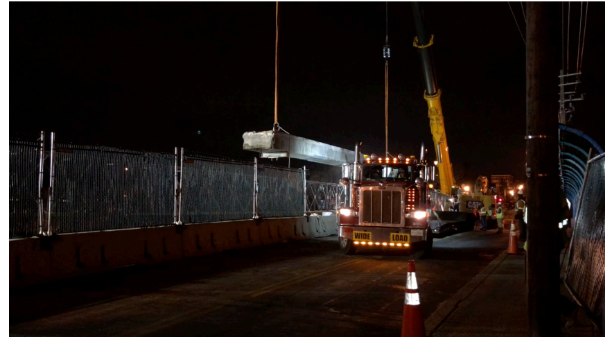
Concrete Beam Removal - Night
